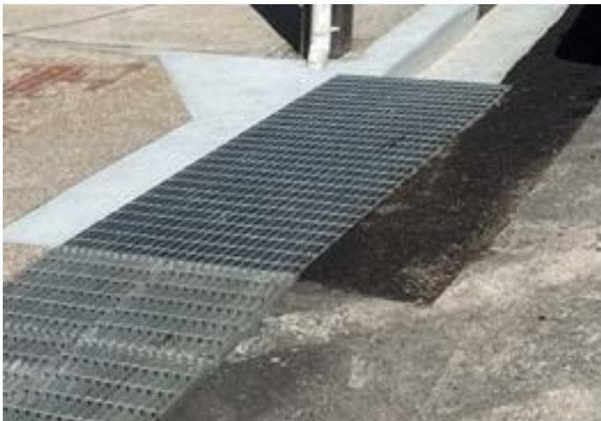
New Grate installed and pipe work directed into pit
