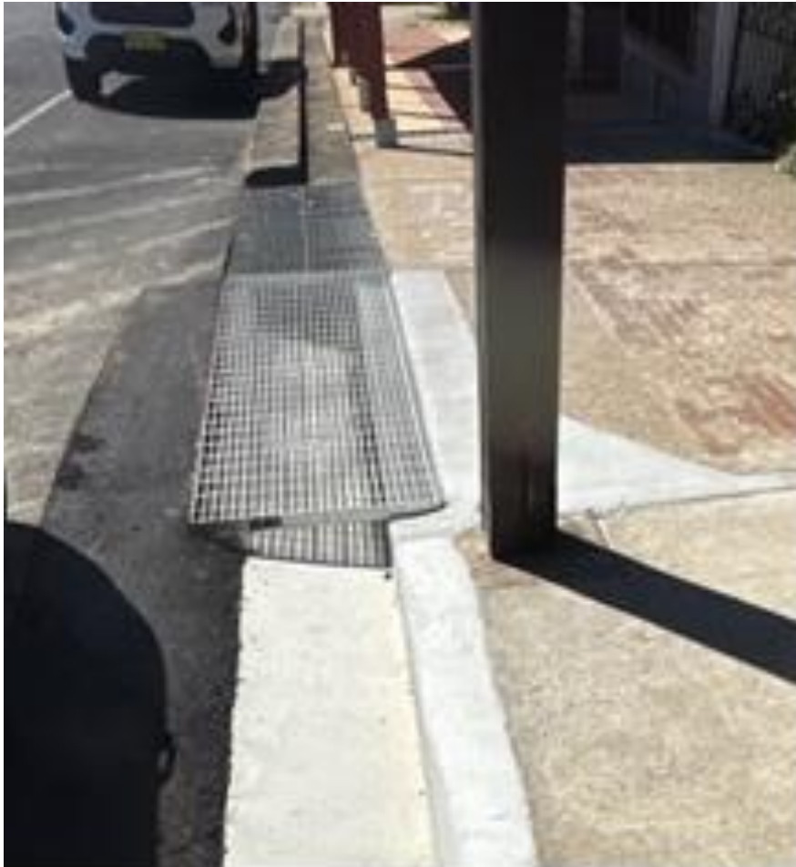
New Grate installed and pipe work directed into pit
