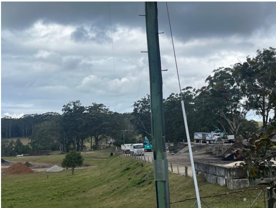
Photo 5 – alignment of 11kV overhead line over yard
