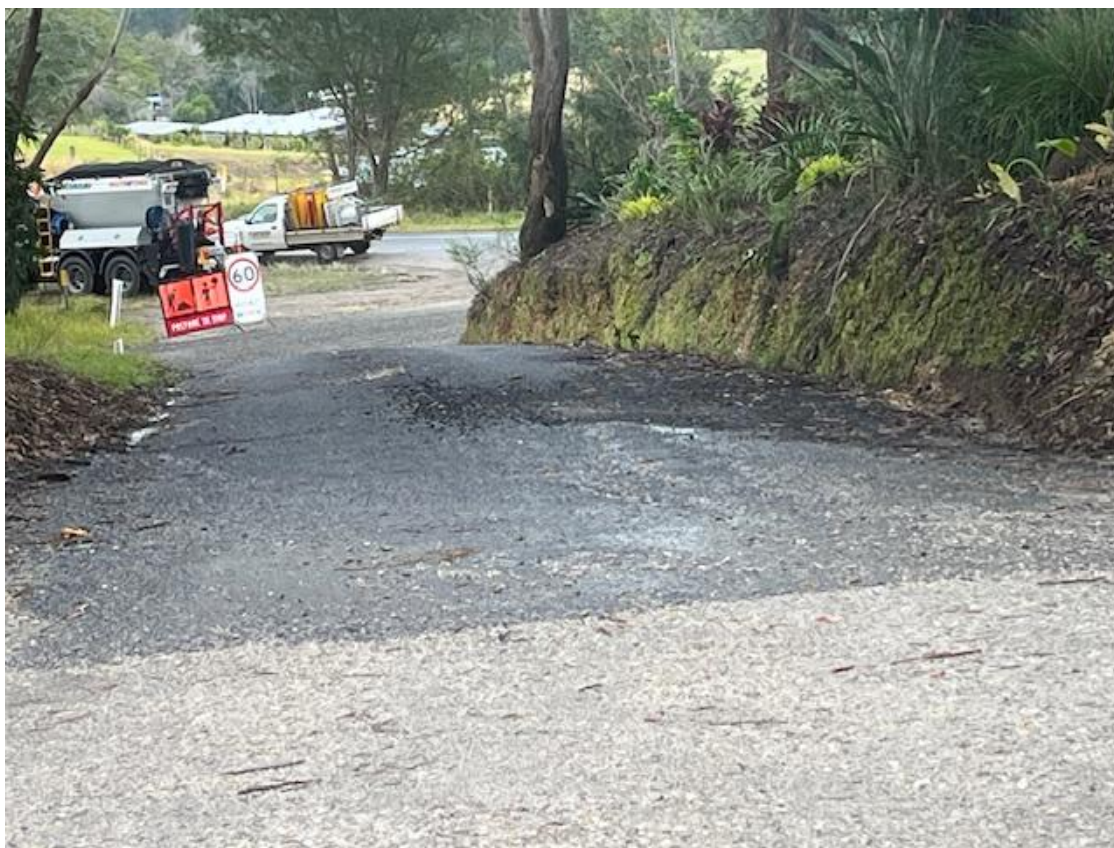
Photo 8 – driveway entrance looking NW with Wirrimbi Road in background
