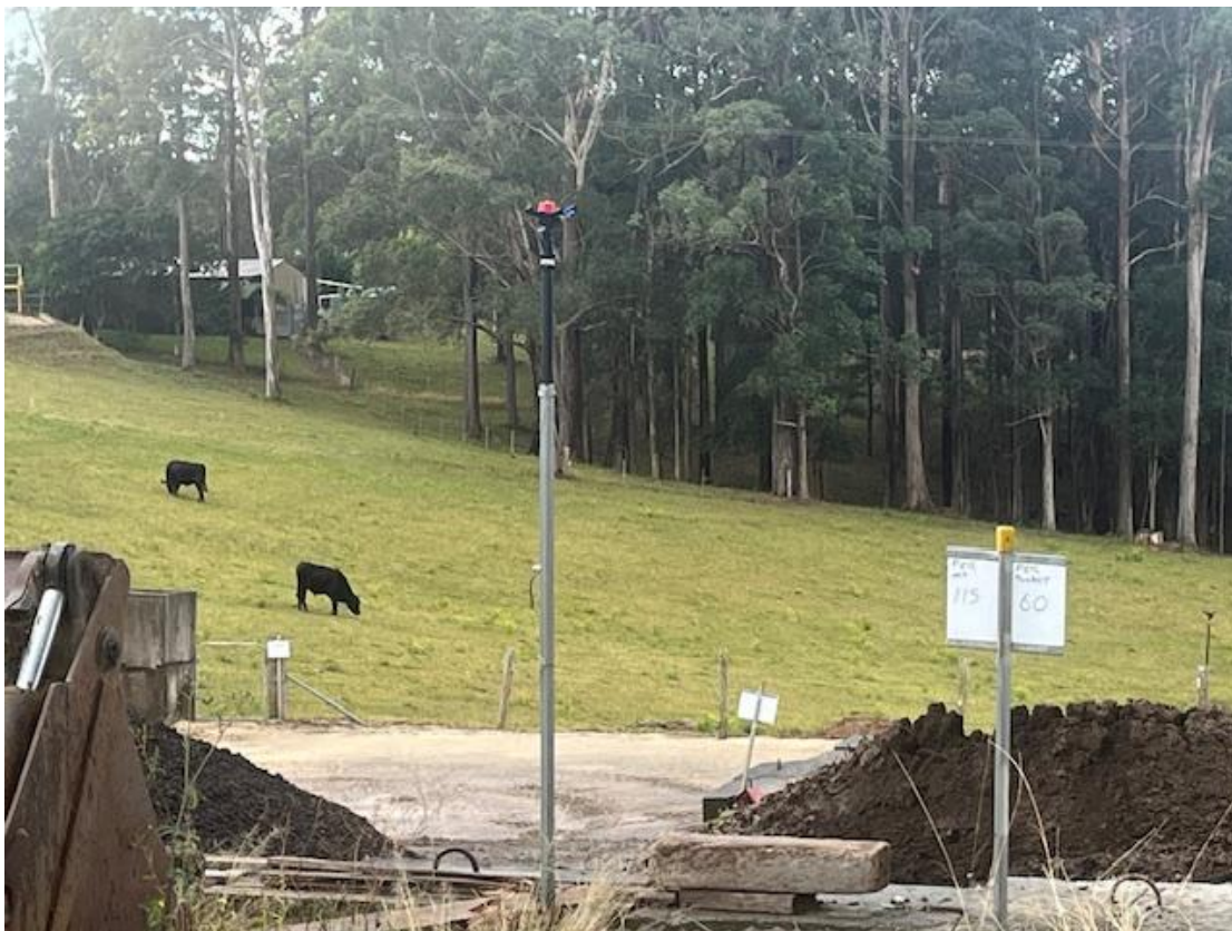
Photo 7 – example of sprinkler head – part of dust suppression system across the yard
