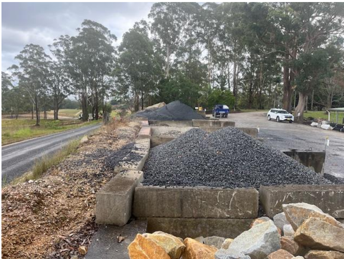
Photo 1 – Aggregate bays on Siding Road reservation with the carriageway to the left
