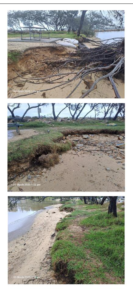
The photo's above show erosion of the area adjacent to the footpath on the small wall behind the V-Wall and along the inner harbour beach side of the reserve.
