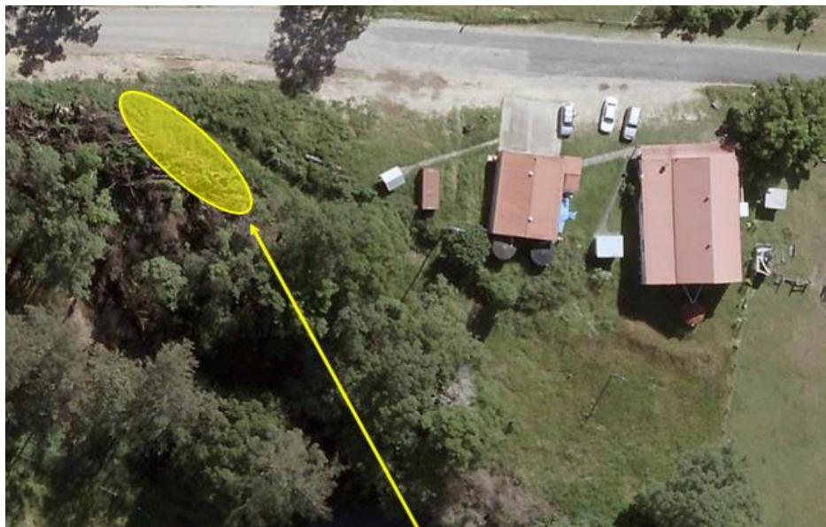
Approximate location of tree debris beside access track to water storage tank and shed (not in aerial photo) South Arm Hall.
